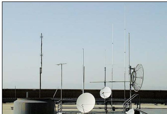
The 445.46 & APRS antenna is the tallest antenna to the right. The 224.70 repeater antenna is the 2-section fiberglass antenna just to the left of the 445.46/APRS antenna.
