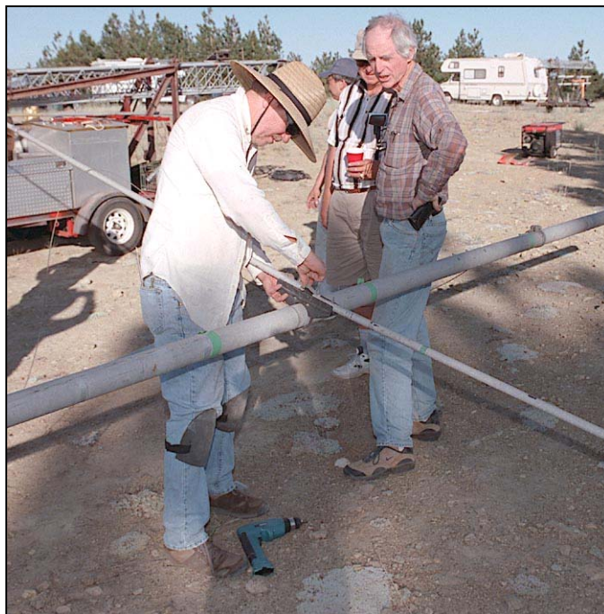
Marty, N6VI, assembling the 20-meter beam
