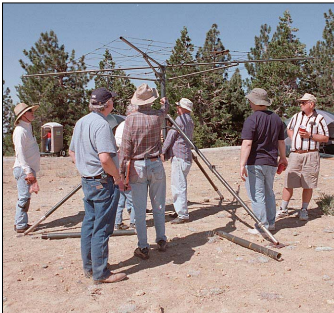
New (for 2002) folding 10 meter-to-6 meter Log Periodic going up
