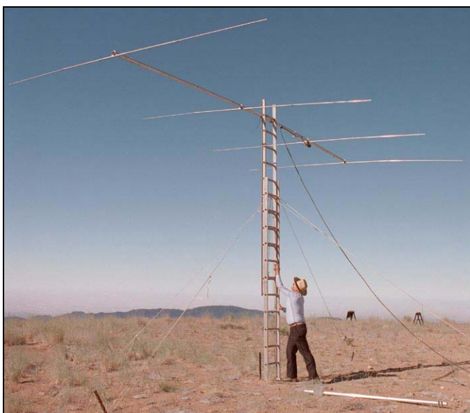
Robb Frederickson, W1EEL, hoists the 10-meter beam on his special Field Day Ladder-Tower
