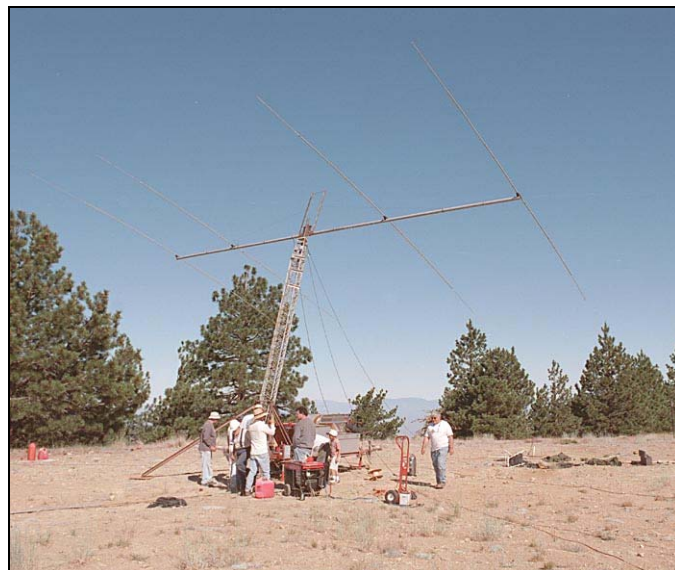
The crew tips the 20-meter beam up on Dave Ritchie's Tower/Generator trailer
