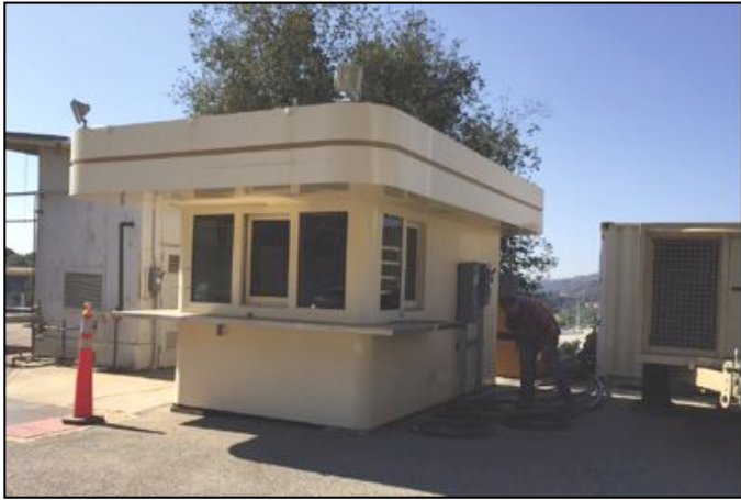
Figure 1: Building 329 - Radio Communications Building (new radio shack). Trailer mounted generator is on the right.
