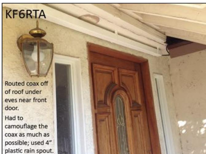
**Figure 5: KF6RTA use of plastic rainspout to camouflage coax**
